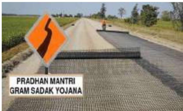
Coir Geotextiles roads in rural areas under PMGSY-III (Representational purpose only)
